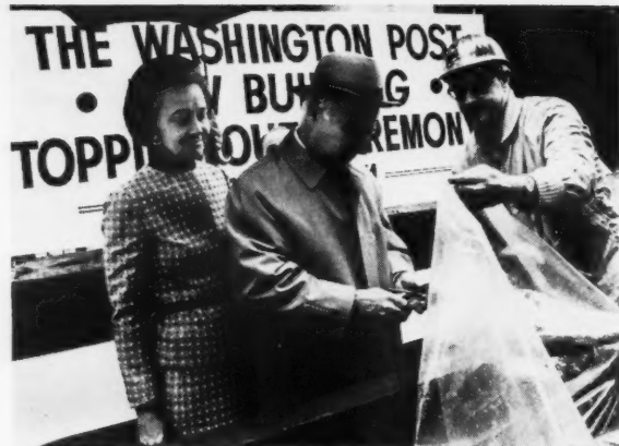
TOPPING OUT—Amid seasonal April showers, Mrs. Katharine Graham, publisher of the Washington Post, looks on as Paul Ignatius, president, is about to autograph the final roof support beam for the newspaper's new half-million square foot addition. Nearly 900 Post employees also autographed the beam before it was raised into place, thus "topping out" the nine-story structure.
